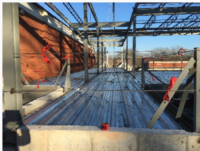
Elevated Decking, Structural Steel Erection, & Exterior Framing
