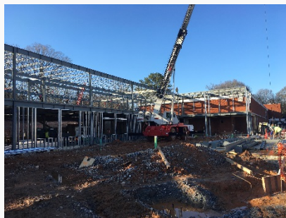
Elevated Decking, Structural Steel Erection, & Exterior Framing
