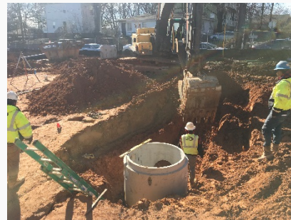
Installation of Yard Inlet Behind Retaining Wall
