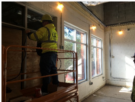
Installation of New Windows/Frames
